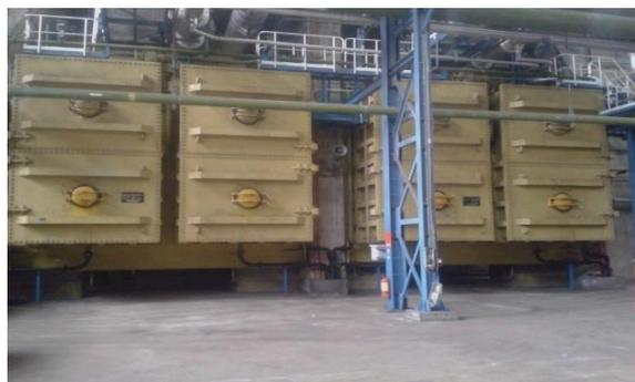
**Gambar 4.** Surface Condensor Unit 1 - 4 PLTU-XYZ
