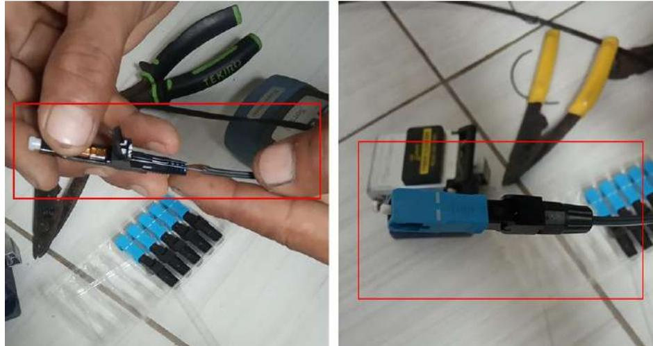
**Gambar 11.** Memasang *Fast Connector*
